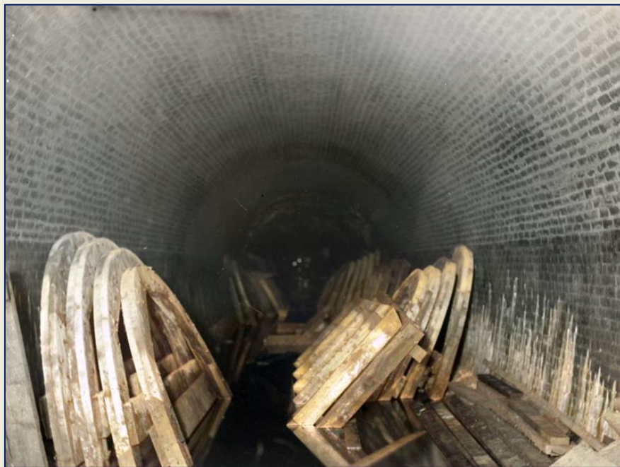
Typical completed section of brick lined tunnel.
