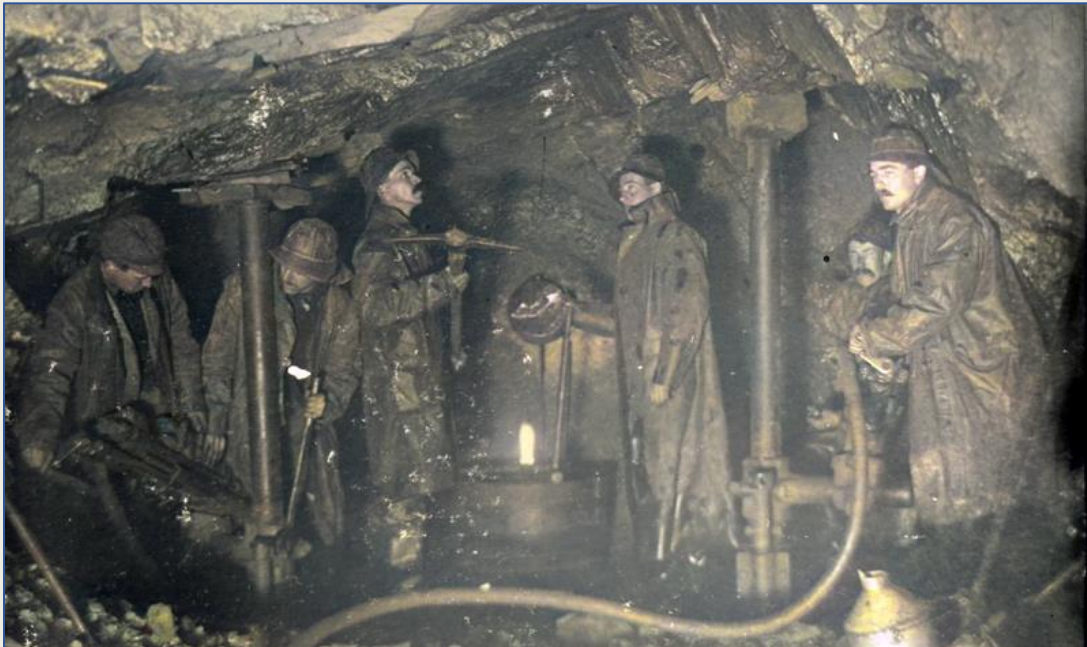
Rock drilling by lamplight.
