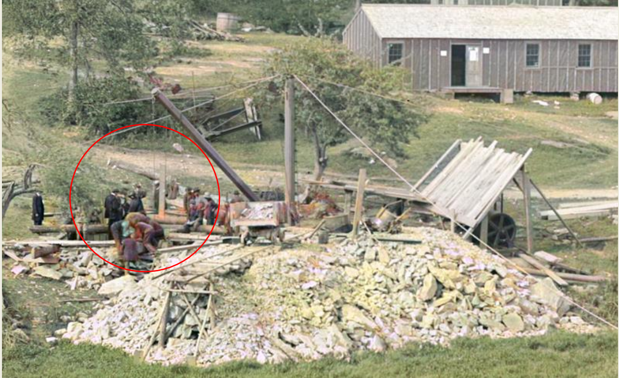
Start of excavation at Shaft No. 3 (circled).
