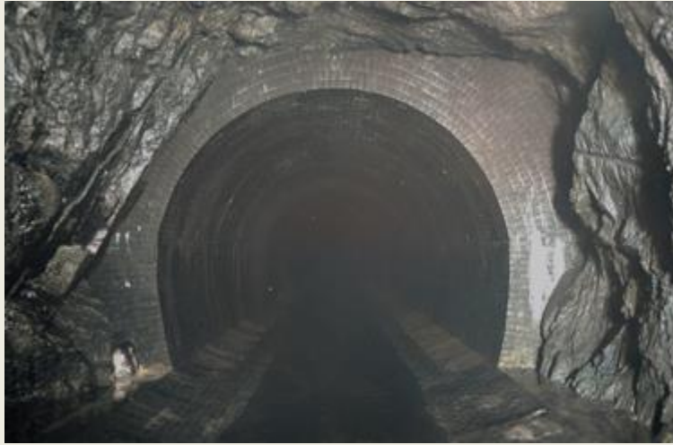
Transition from unlined rock to brick lined tunnel.
