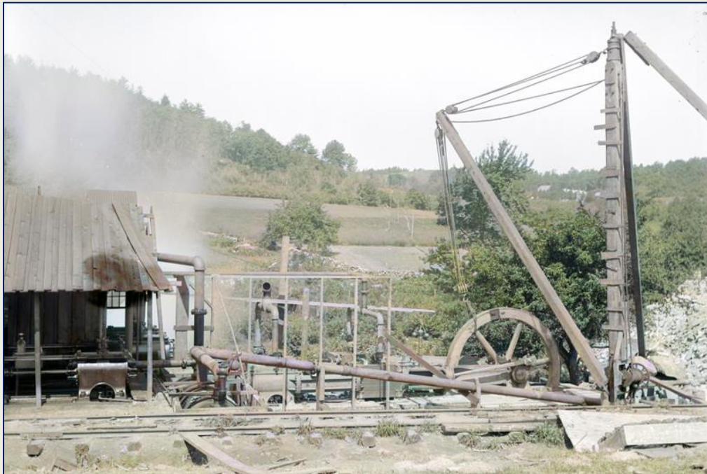
Compressor at Shaft No. 4, from the east.
