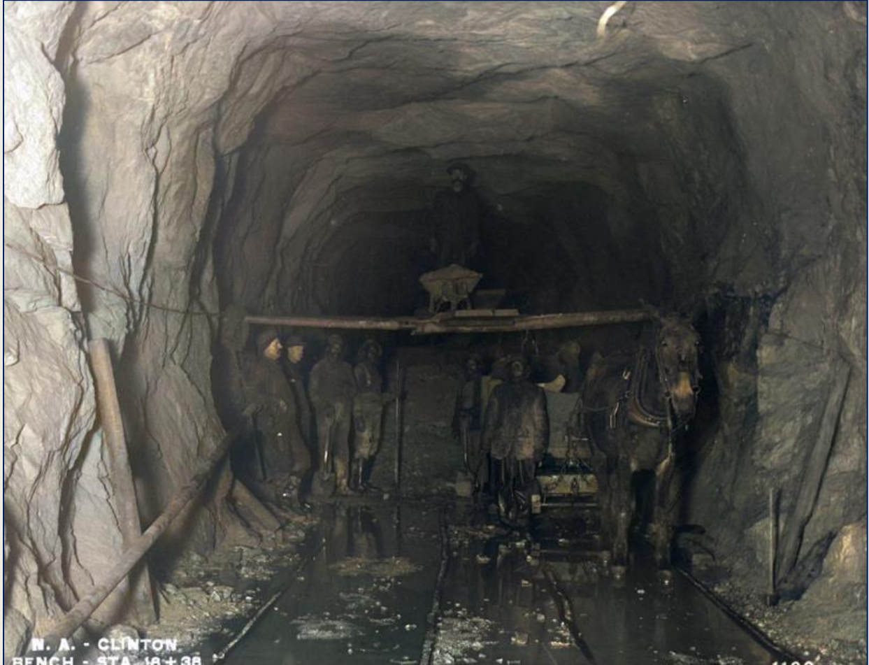
Excavating at a typical rock face.
