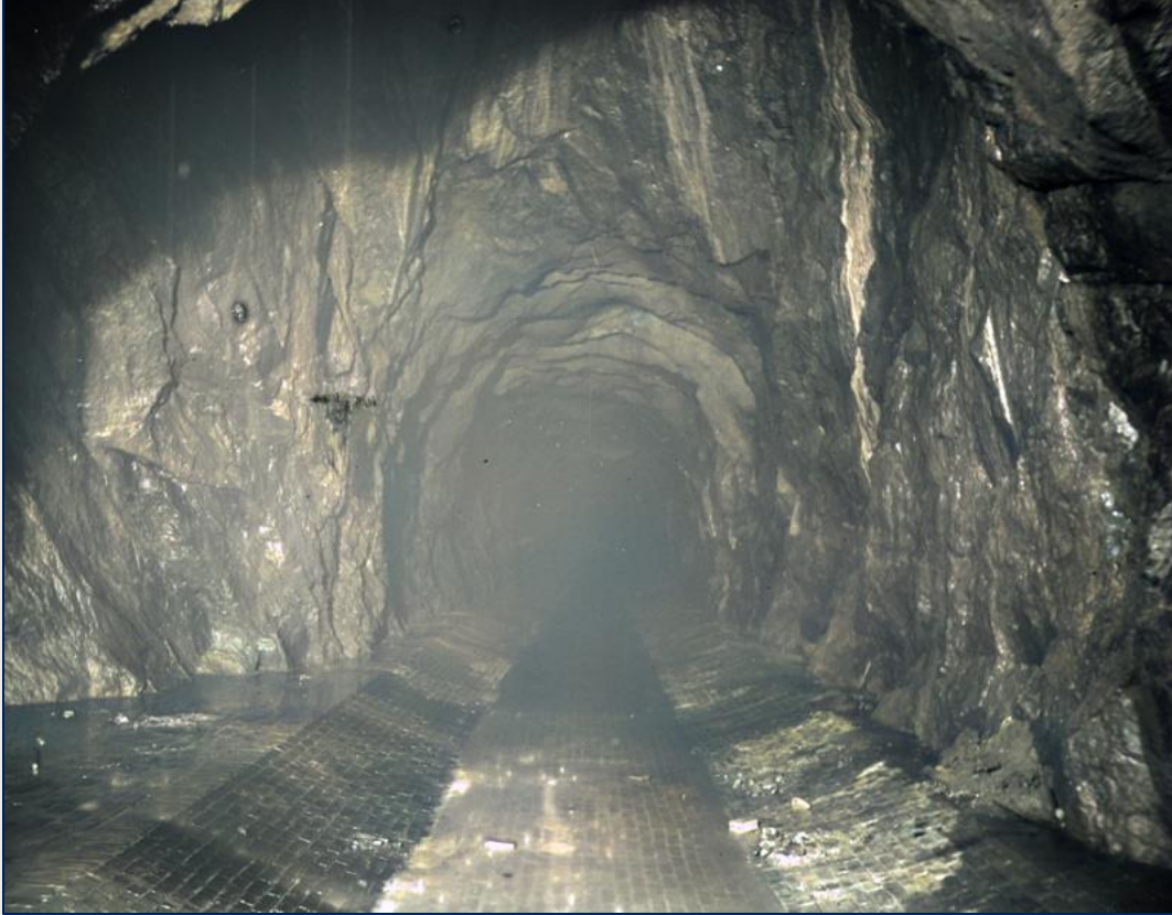
Section of tunnel below Shaft No. 2, in rock with brick invert.
