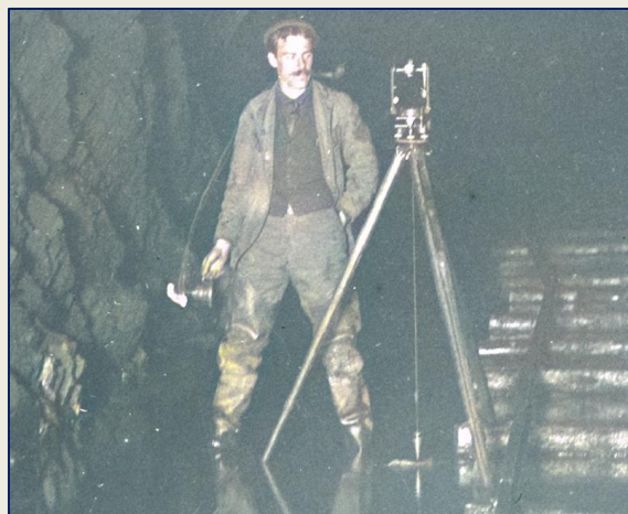
Surveyor in the tunnel with rubber boots, hand lamp and pipe.
