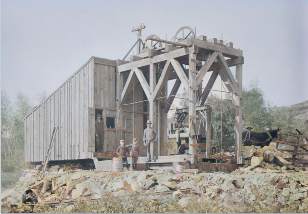
Headhouse at Shaft No. 2.
