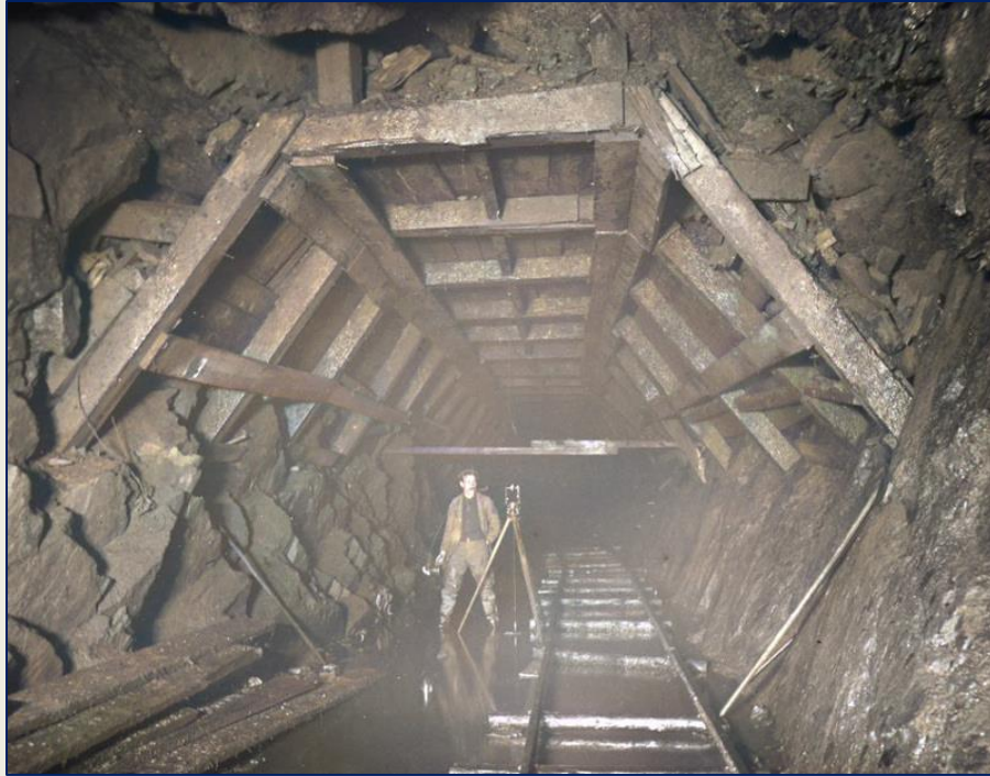
Surveyor with transit inside a partially completed tunnel.
