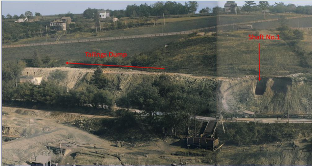
Shaft No. 1 tailings dump along River Street.
