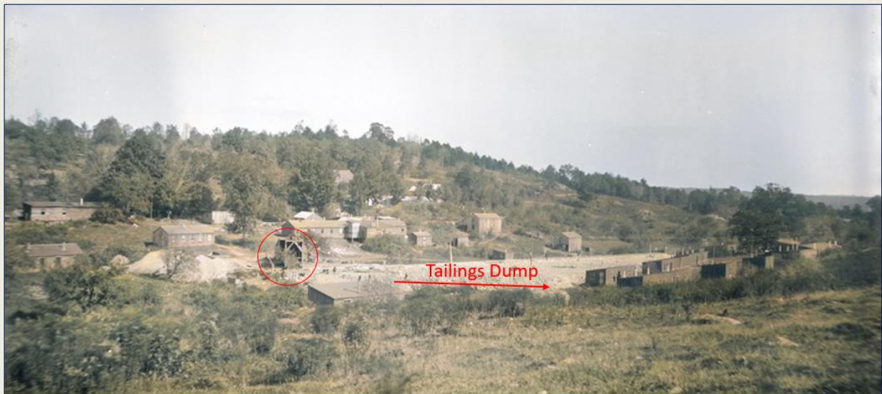
Shaft No. 3, contractor's headquarters and labor camp.
