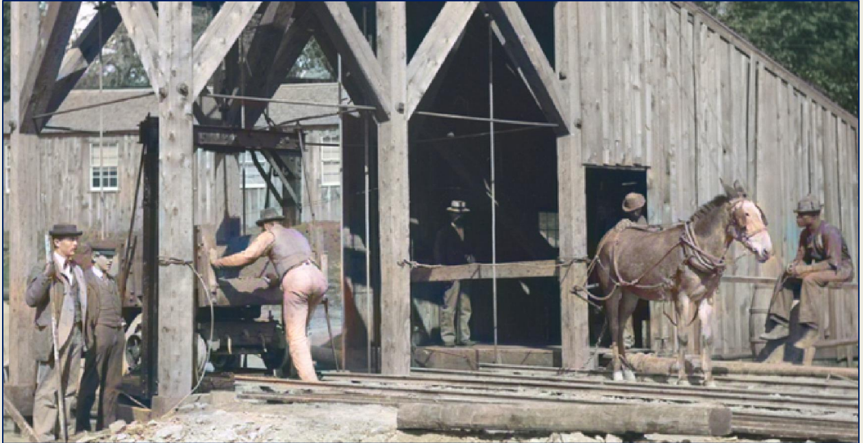
Headhouse at Shaft No. 3.
