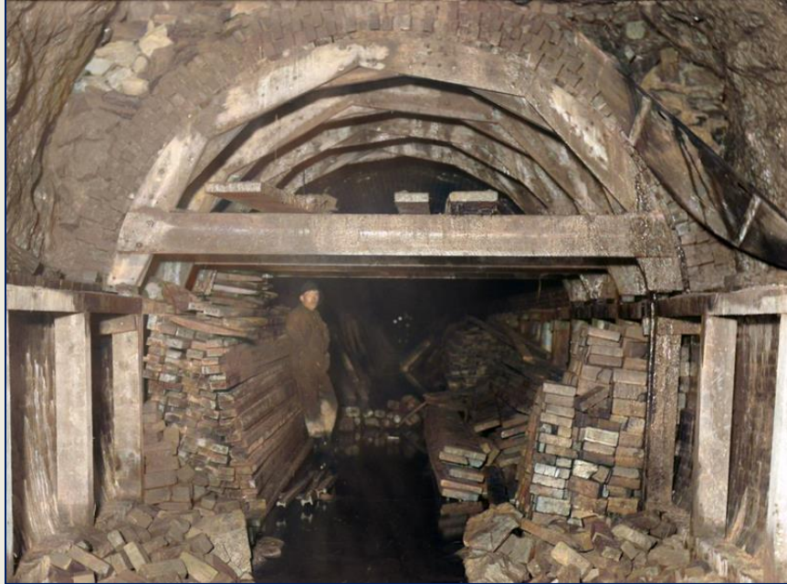
Brick liner on entire perimeter.
