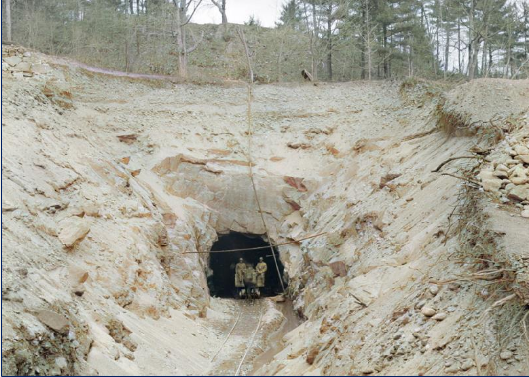
Driver and horse dumping tailings from the Portal, April 27, 1897.
