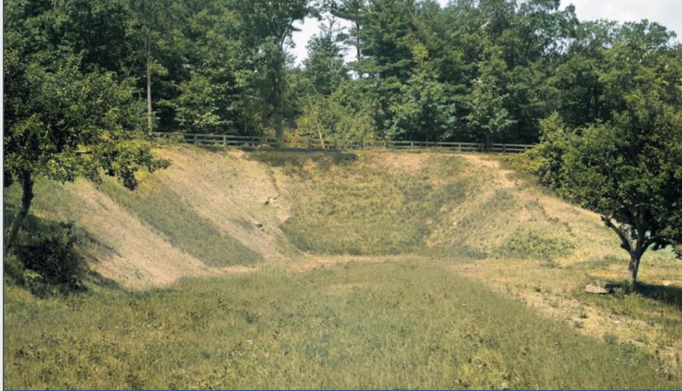
The tunnel Portal at Derby Road.
