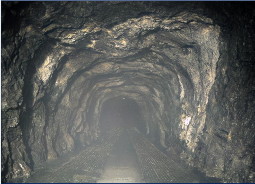
Section of tunnel in rock with brick invert.
