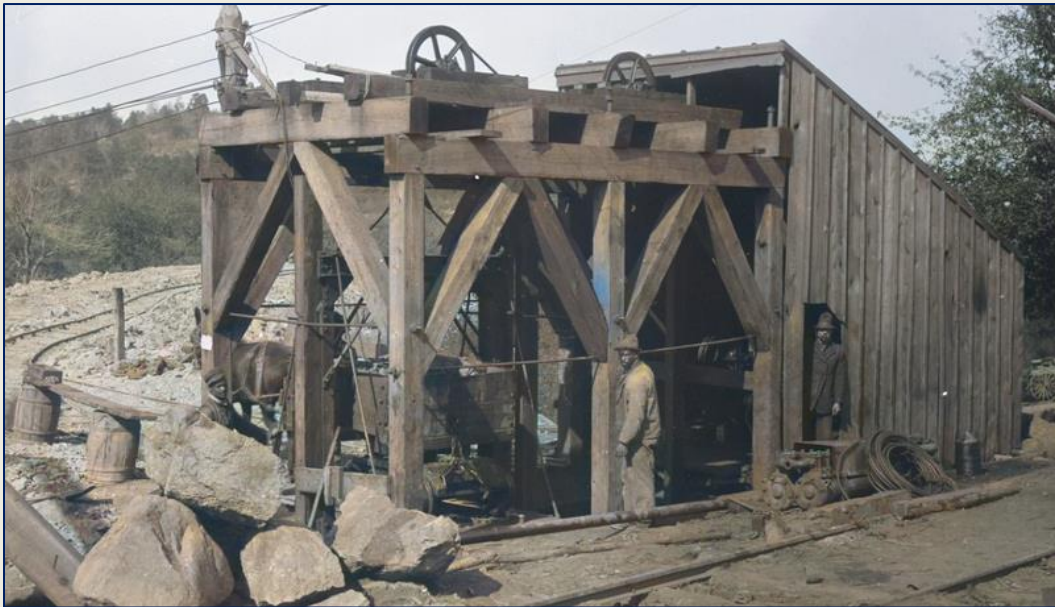
Headhouse at Shaft No. 4.
