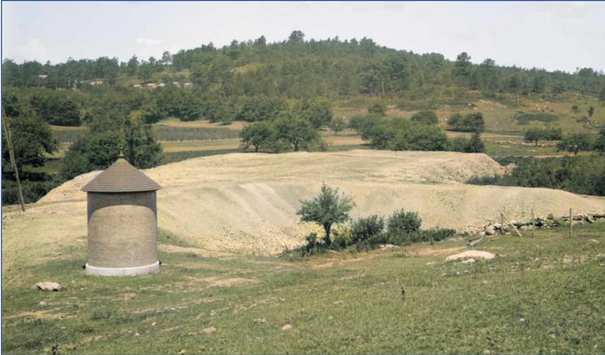
Final cleanup of Shaft No.4 site.
