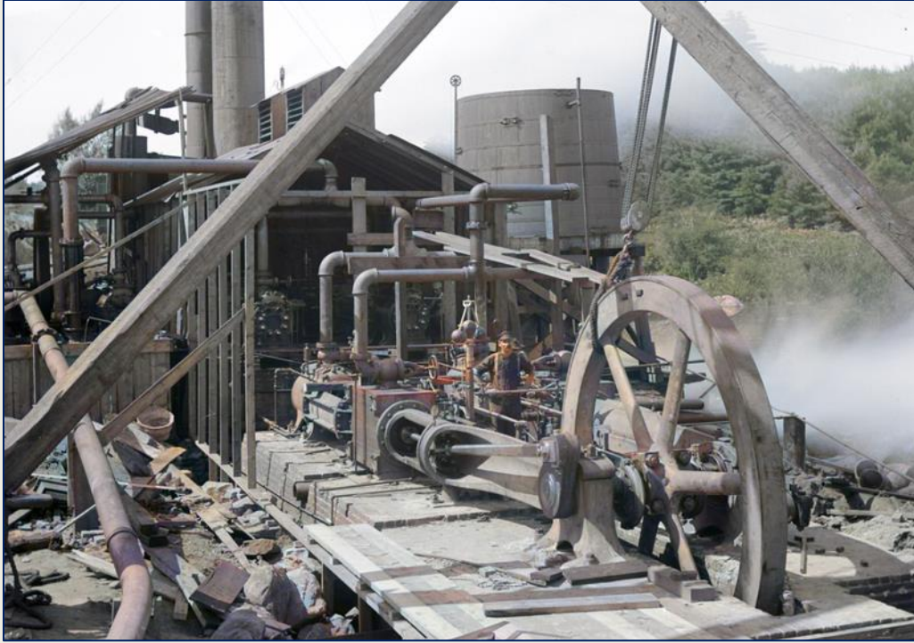
Installing compressor flywheel at Shaft No. 4, from the east.
