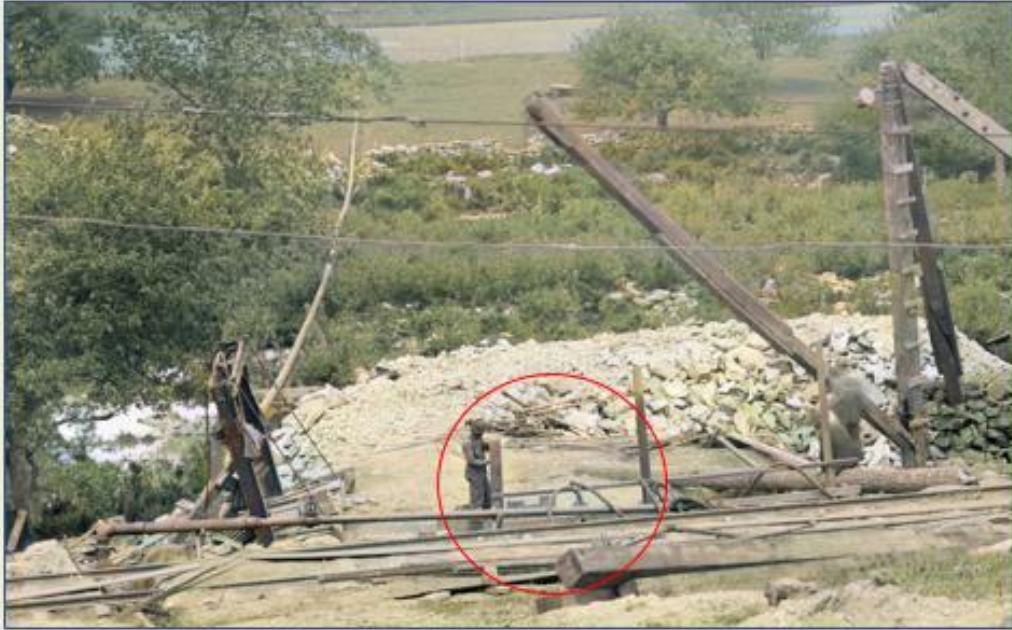
Start of excavation for Shaft No. 2 (circled).
