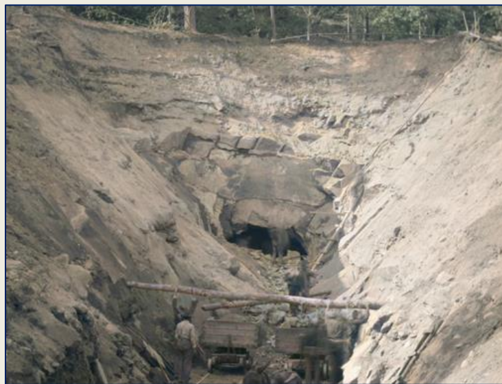
The Portal approach excavation to the tunnel.
