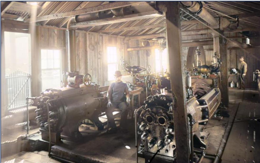
West compressor plant.
