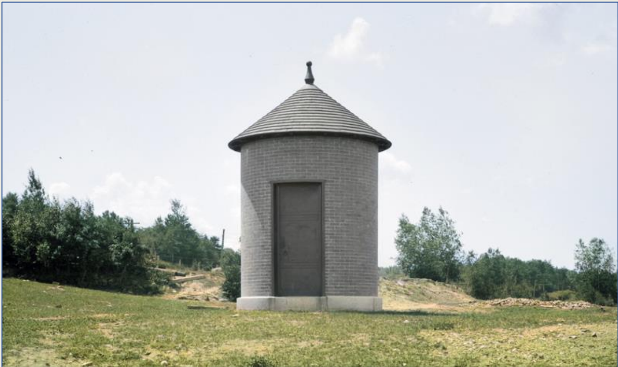
On the top of the shaft a small, circular gray brick house was built to facilitate access to the tunnel.
