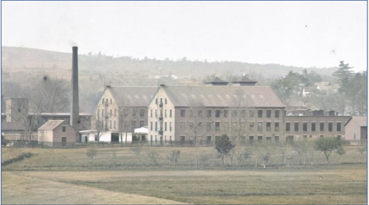
Clarendon Mills was the second largest mill in the valley, employing around 200 workers.
