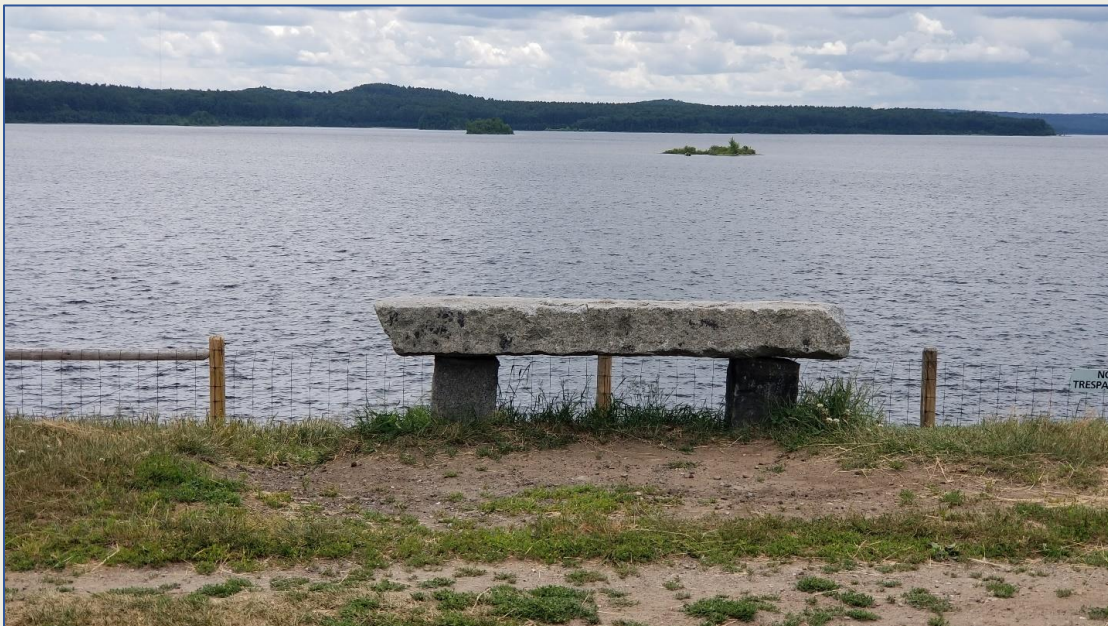
Sandy Pond, looking west from North Dike.
