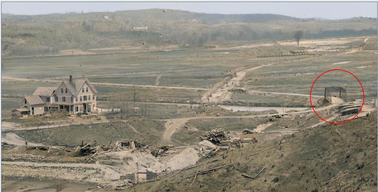
Scar Bridge and drained millpond. Beyond soil removal tracks lead off to the North Dike.
