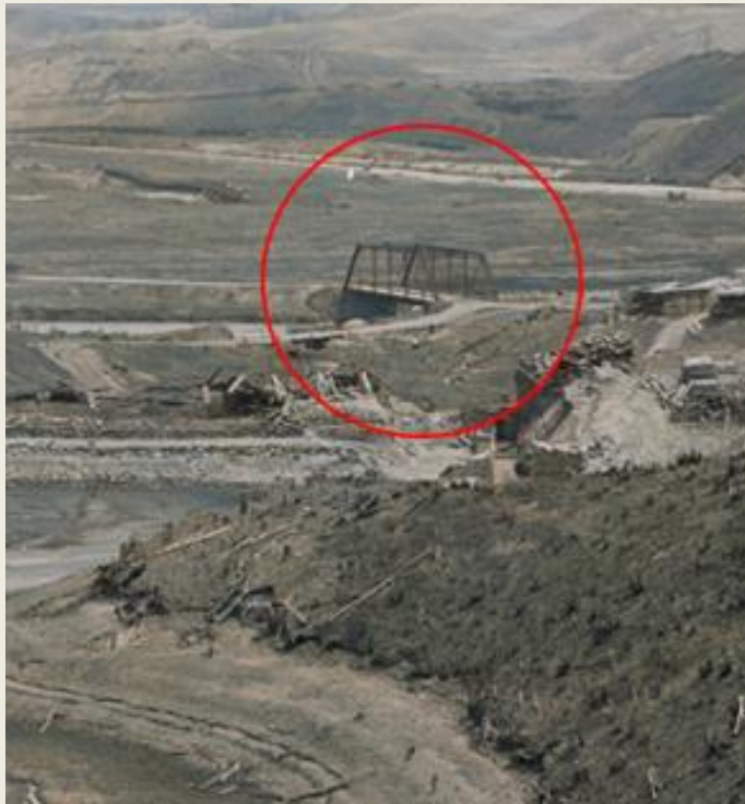
Scar Bridge spanning the Nashua River near the drained millpond.
