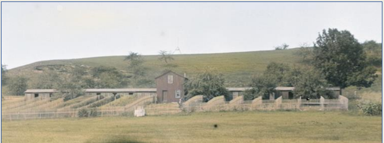
Fifteen bay hennery with center feed shed.
