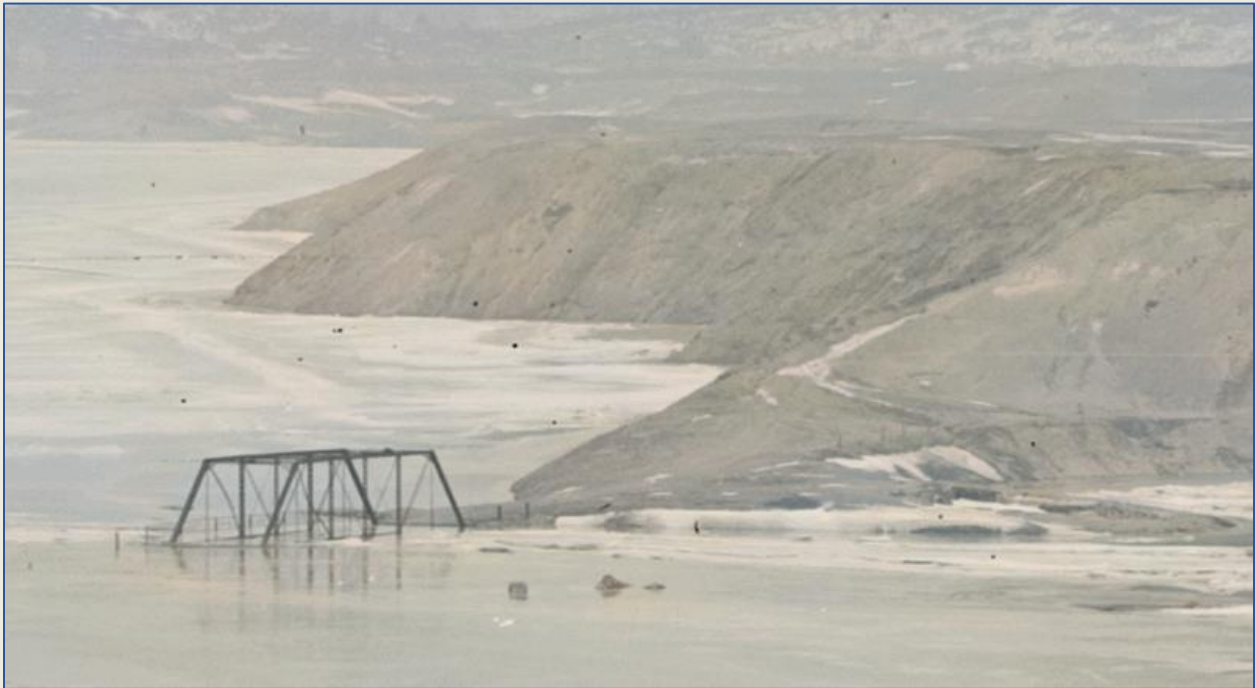
Houses and buildings removed, the carriage bridge was left standing in place.
