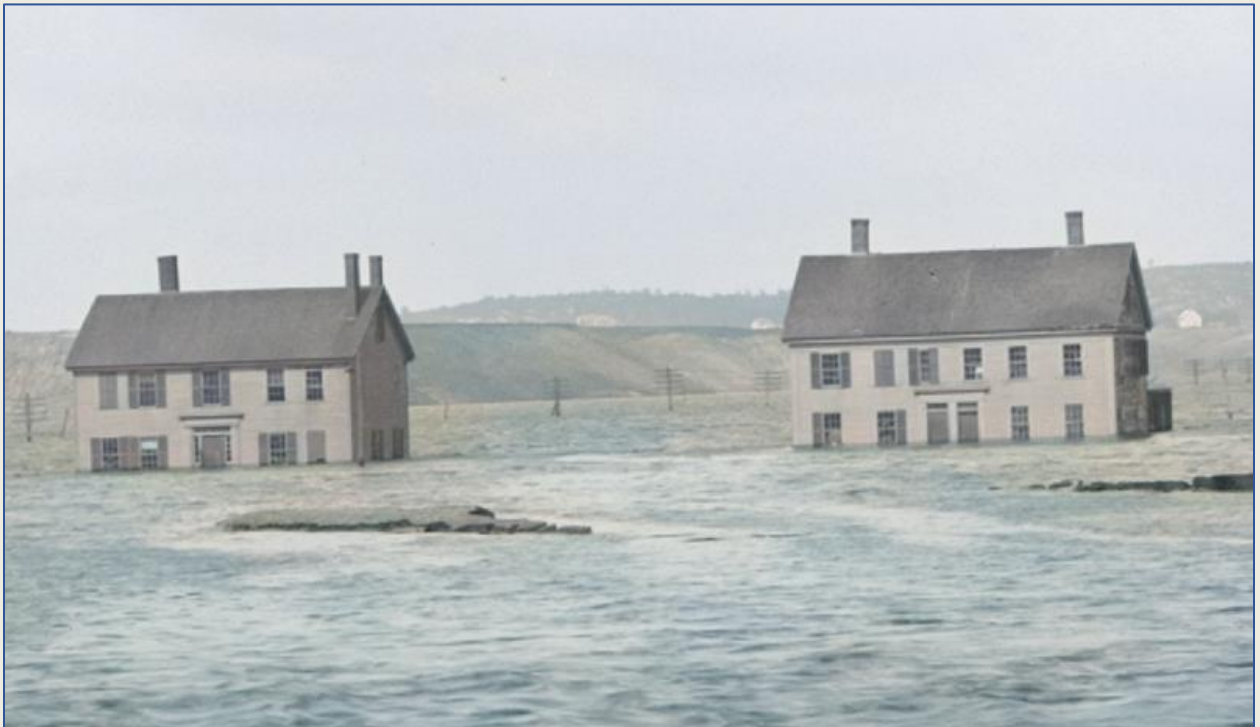
Foremen's housing on the mill property.
