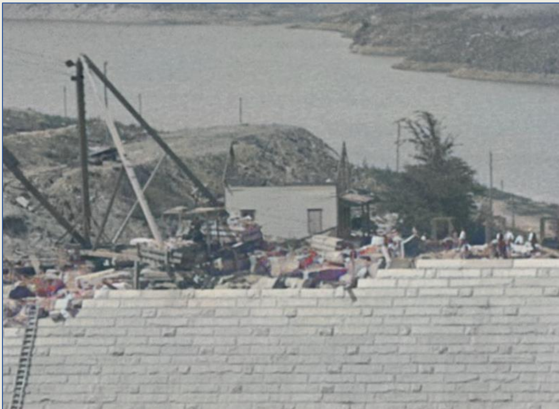
Ultimately both houses were demolished.
