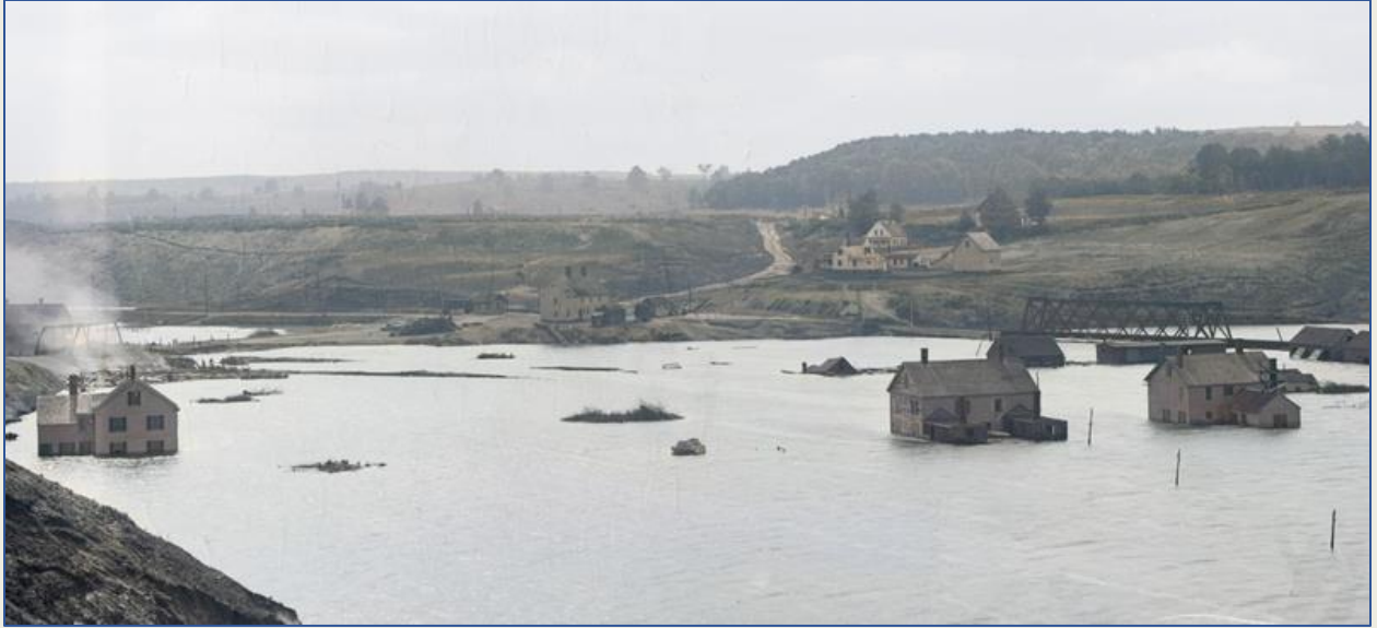
Mill housing, bridges and local residences. June 22, 1903
