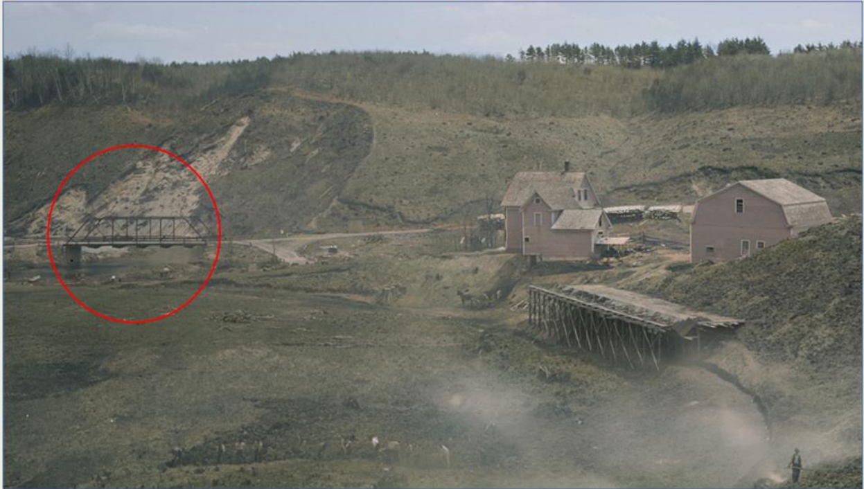
Scar Bridge near Albertson's sawmill and topsoil dumping platform.
