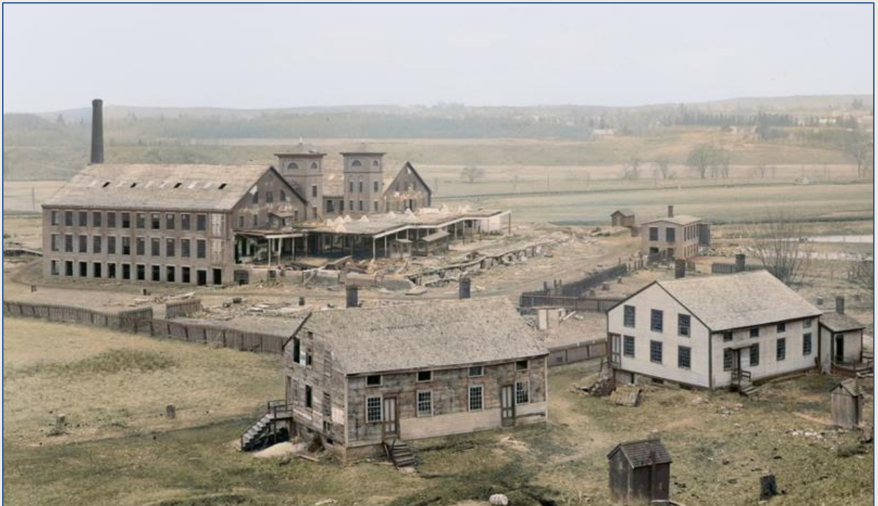
Clarendon Mills under demolition. April 8, 1902
