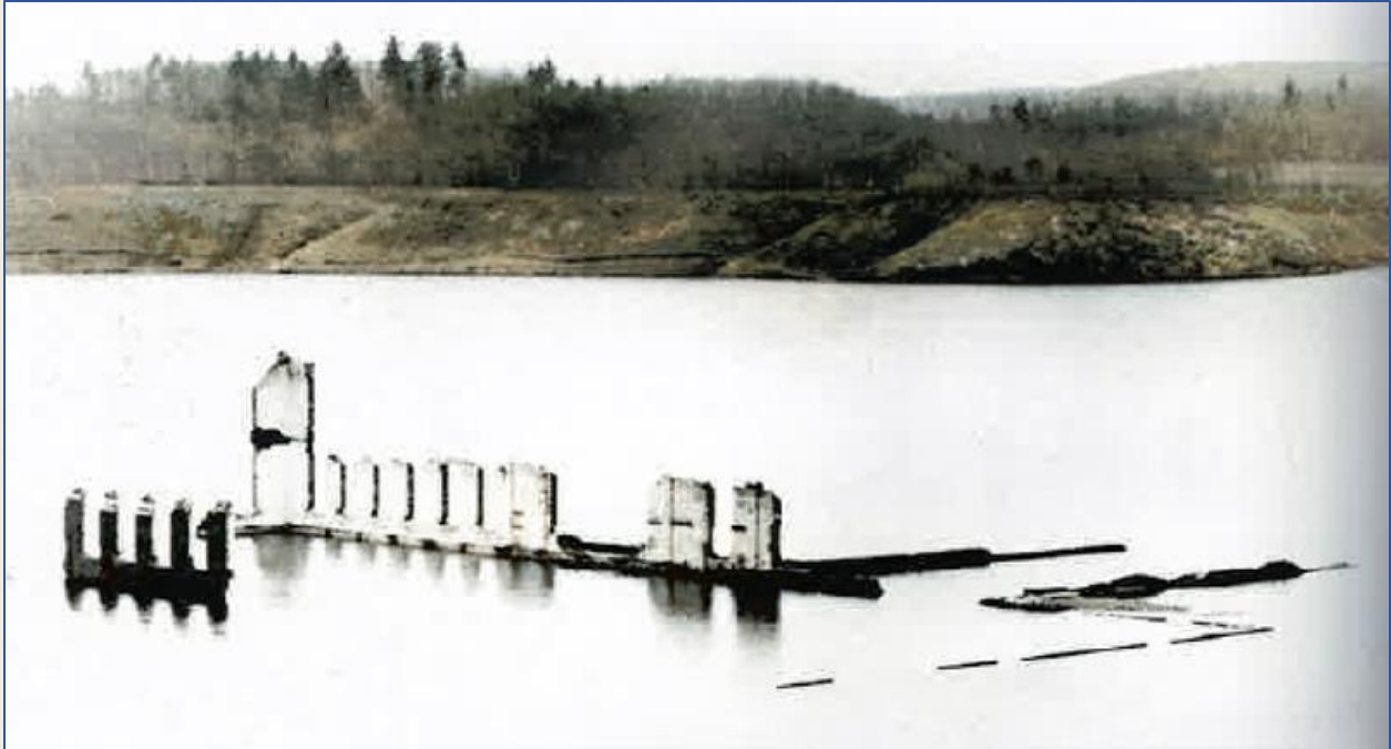
So it remains today, with the top of the brick wall barely twenty feet below the surface.
