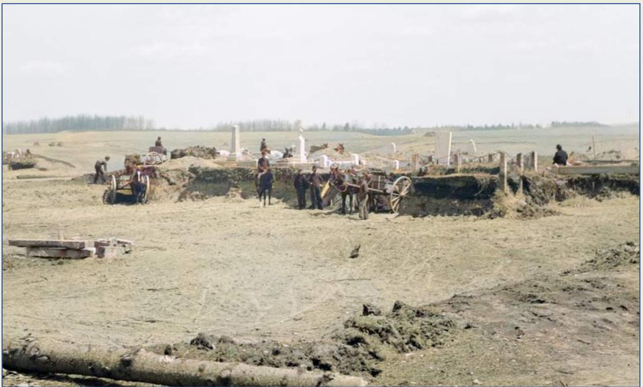
As the graves were removed the good quality gravel was taken for use in the North Dike.
